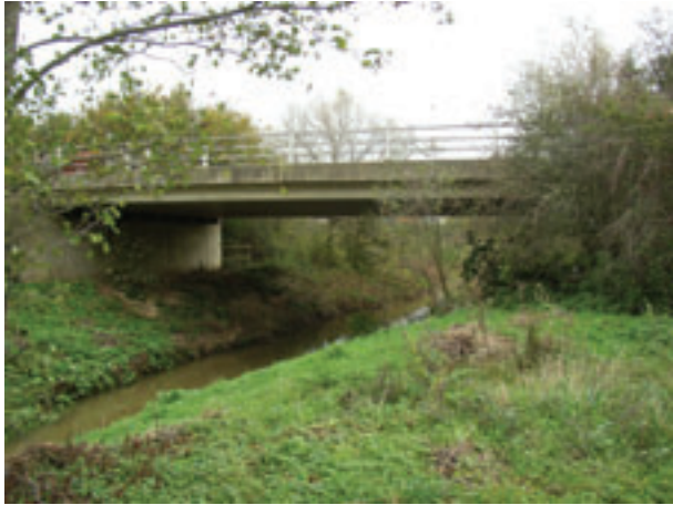
River Uck Bridge, A22
