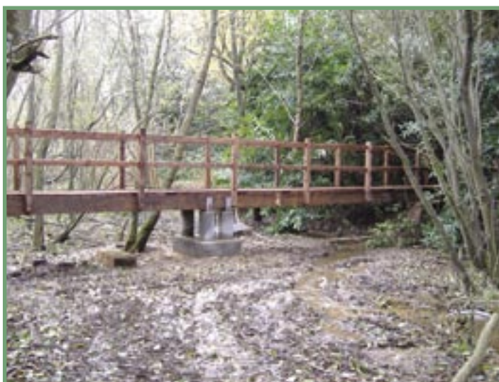
New footbridge on Warbleton footpath 15
