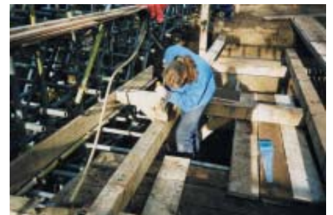
Work on the new bridge
