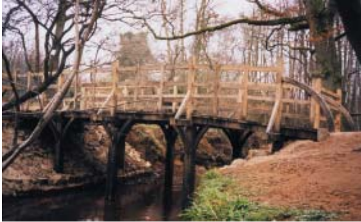
The new Pooh Bridge
