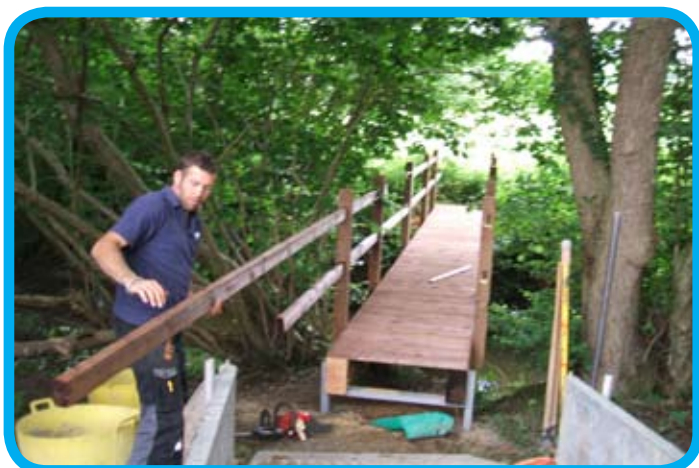
Karl Woolmer installing a hand rail on a new bridge.
