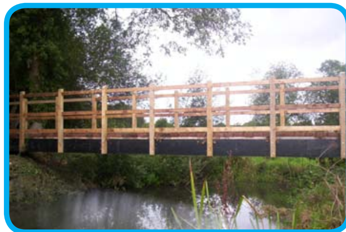
Overs Bridge, Barcombe
