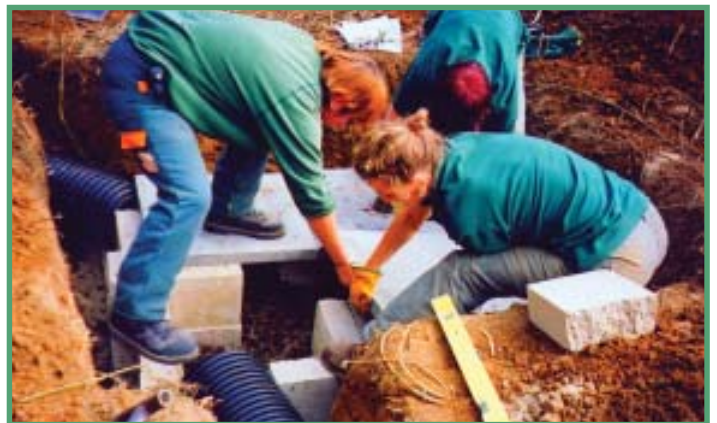
Helping out otters – building an otter holt
