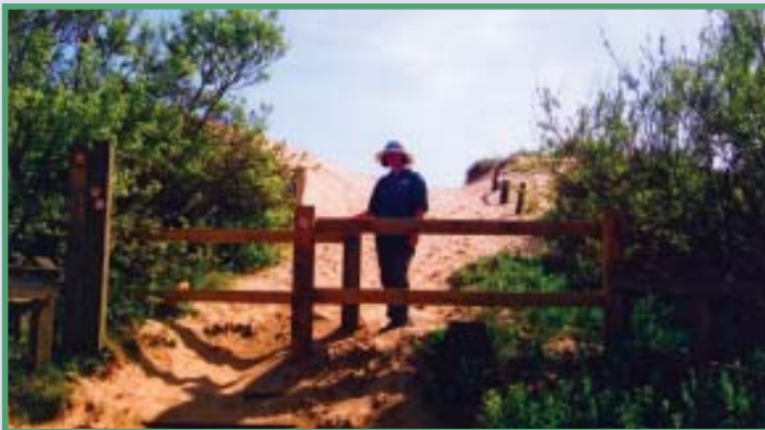
New barriers installed at Camber
