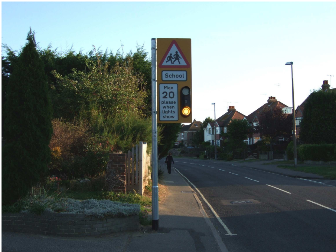
Photo 2 – flashing amber beacons (West Sussex)
