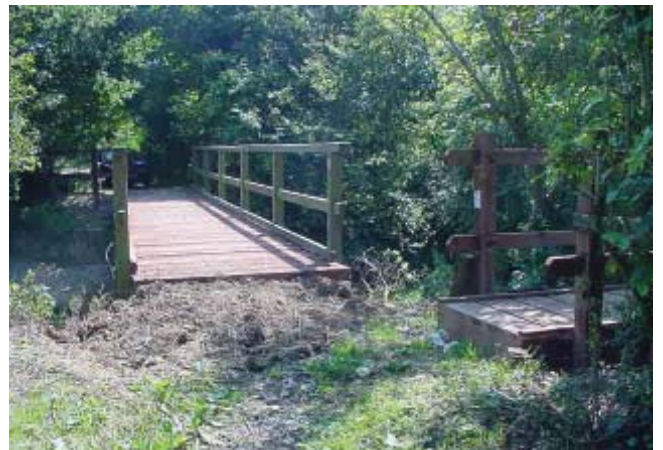
The new Sessingham bridge and nearby footbridge
