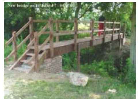
New bridge near Isfield church
