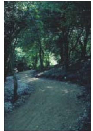
Resurfacing work at Bunkershill Plantation
